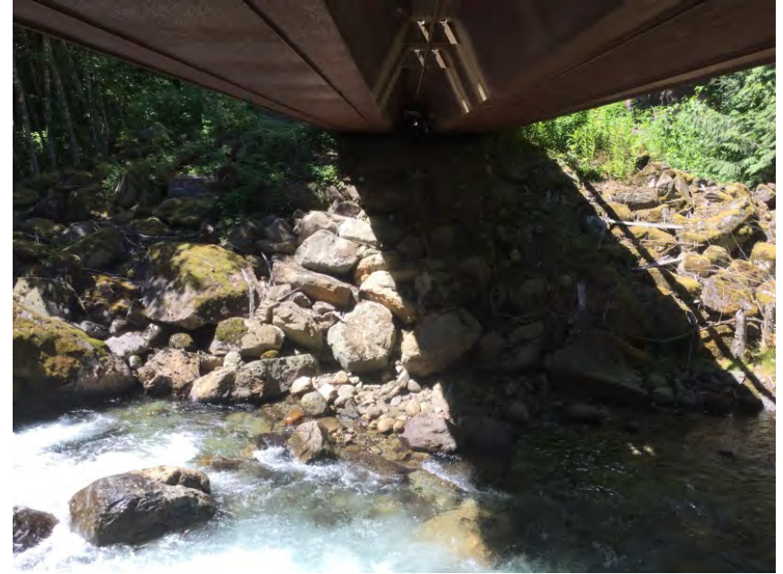
Left Bank Abutment when facing downstream
