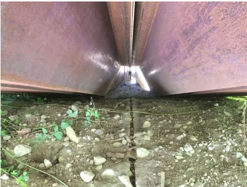
Left Bank Abutment when facing downstream
