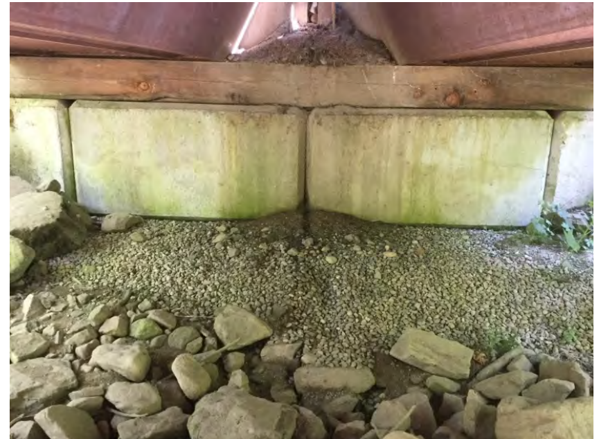
Right Bank Abutment when facing downstream
