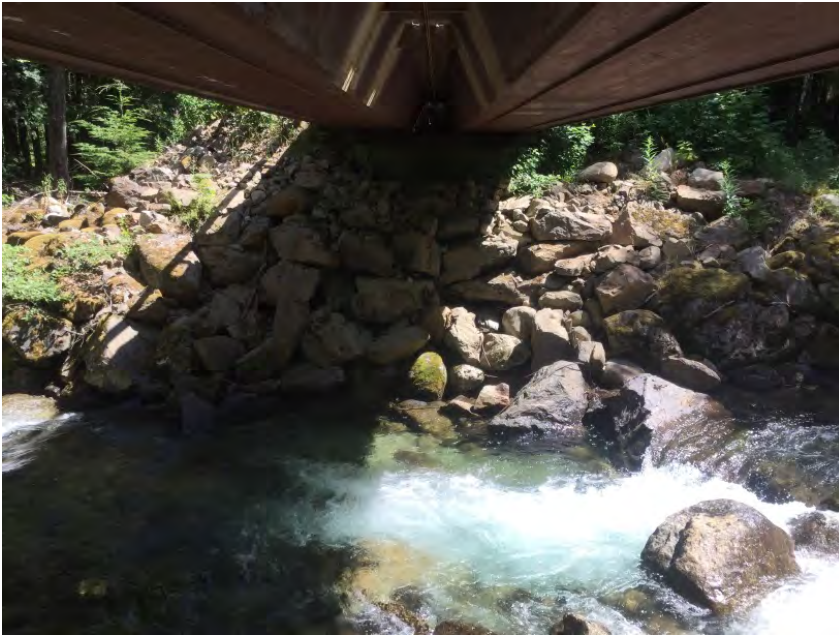
Right Bank Abutment when facing downstream
